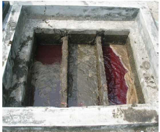
Figure 4. The wastewater (mostly containing oil and grease) from the drain was collected in this concrete solid trap compartment.
